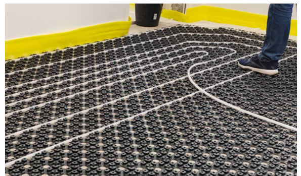
Fastening underfloor heating pipe in LOWTOP castellated mat
