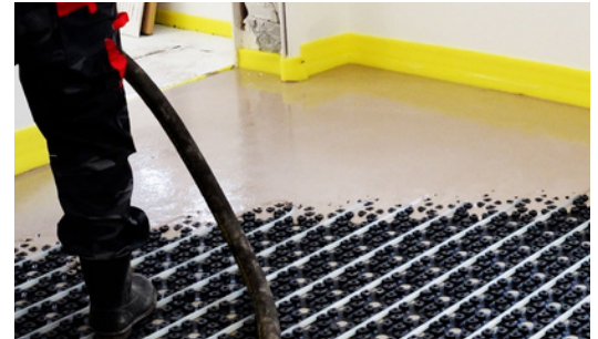
Flooding the underfloor heating system self-leveling mass
